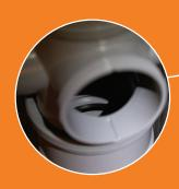
Expansion gap can be inspected by the installer and Building Control Officer when installed with an Access Pipe fitting.
