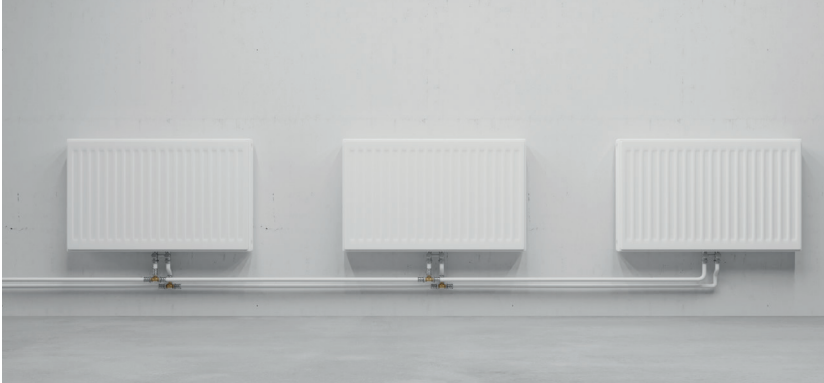
Fig. 46: Double pipe radiator heating.
