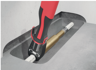
Fig. 30: Installation steps repair coupler.
