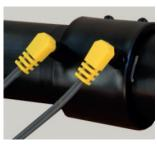
12. During and after fusion, check the message on the display of the fusion unit. When the fusion is successful, remove the fusion cables. Check the fusion indicators on the coupler. Both indicators have to be visible. If not, the coupler must be cut out and a new coupler should be installed. Defective connections must not be welded twice!
