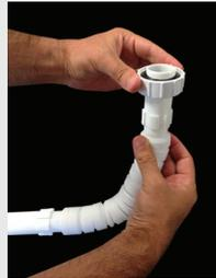
2- Remove the outlet side union of the HepvO and connect the below hose.
