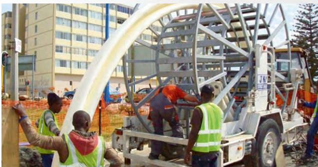
South Africa, Durban, DN250, sewer rehabs
