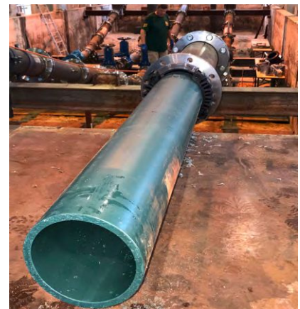
Installation Compact Pipe®, DN200, SDR 17, PE 100 at the IKT Warentest challenge
