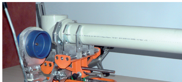
finished weld after the cool-down
