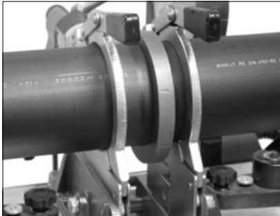
Heating with the heating plate
