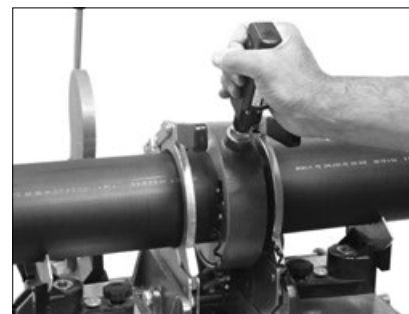
Planing the pipe ends
