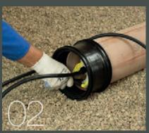
Fit expanding stoppers in the end of all pipelines and branches
