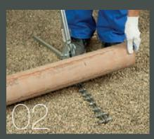
Pass the chain under the pipe, aligning the cutting wheels with the desired cut line
