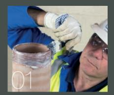
Lubricate the pipe end
