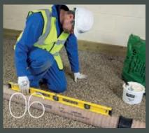
Check the pipeline is laid to the correct gradient
