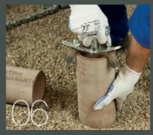
Remove any sharp edges with pipe trimmer
