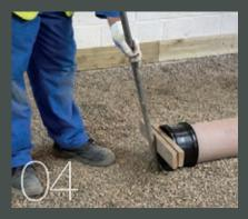
Larger pipe sizes can be jointed with the assistance of a bar
