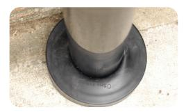
downpipes into below ground drainage:
