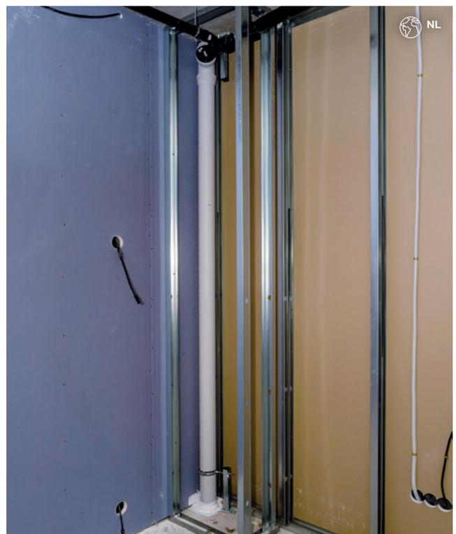
Figure 12: Drywall walls with fastening via brackets to ceiling and floor
