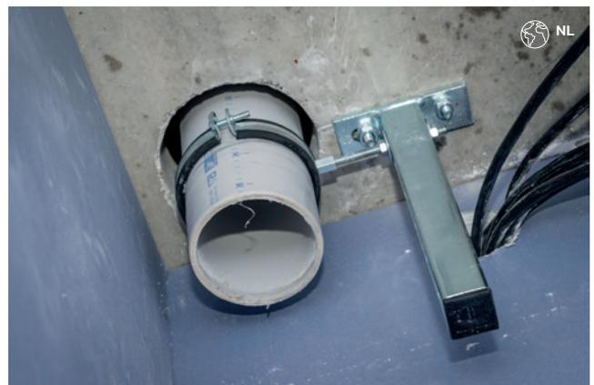
Figure 11: Fastening to elements containing mass
