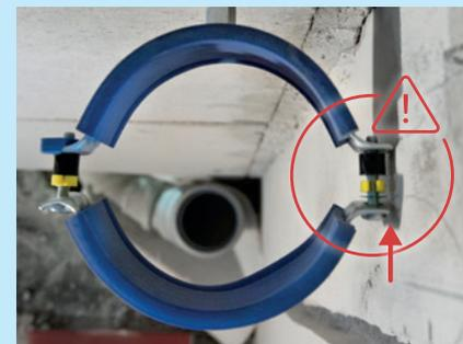
**Figure 40:** Aligning the pipe brackets correctly
