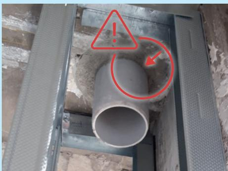
Figure 20: Forgotten structure-borne sound decoupling
