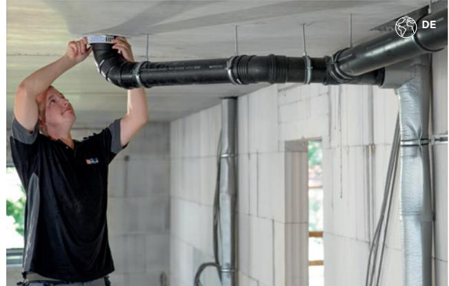
**Figure 39:** Wastewater pipe with sound insulation hose
