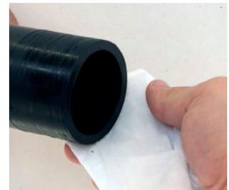
6. Clean the peeled area of the pipe with HDPE cleaner using a clean, lint-free, colourless cloth in a circumferential direction and let the cleaner evaporate.
