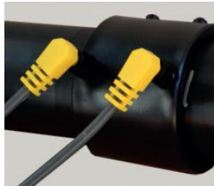
12. During and after fusion, check the message on the display of the fusion unit. When the fusion is successful, remove the fusion cables. Check the fusion indicators on the coupler. Both indicators have to be visible. If not, the coupler must be cut out and a new coupler should be installed. Defective connections must not be welded twice!
