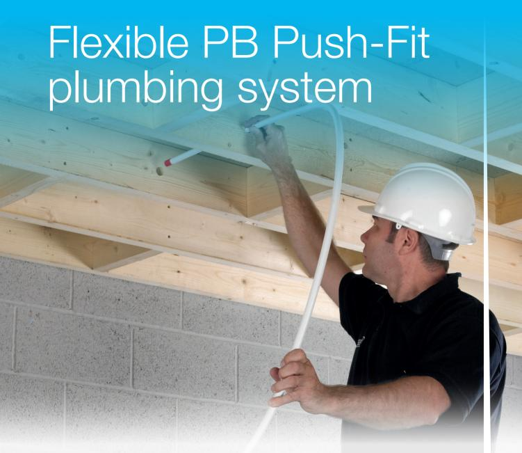
Hep20® is the professional polybutylene (PB) pushfit plumbing system for hot and cold water and central heating. It offers a fully comprehensive range of white fittings and unique features designed to reduce installation time and improve operating performance:
