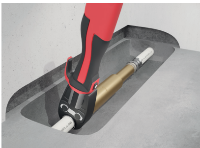
Fig. 30: Installation steps repair coupler.
