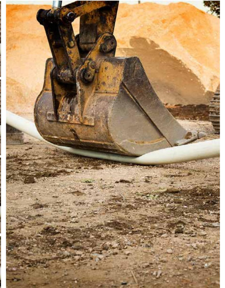
Because of the high flexibility of Apollo O-PVC it can be applied up to 11° without using elbow. So, fewer fittings are used. Apollo pipes can be used with socketed U-PVC and cast iron fittings. The important point is that the pipe needs to be entered to the socket completely. (See the User manual section)
