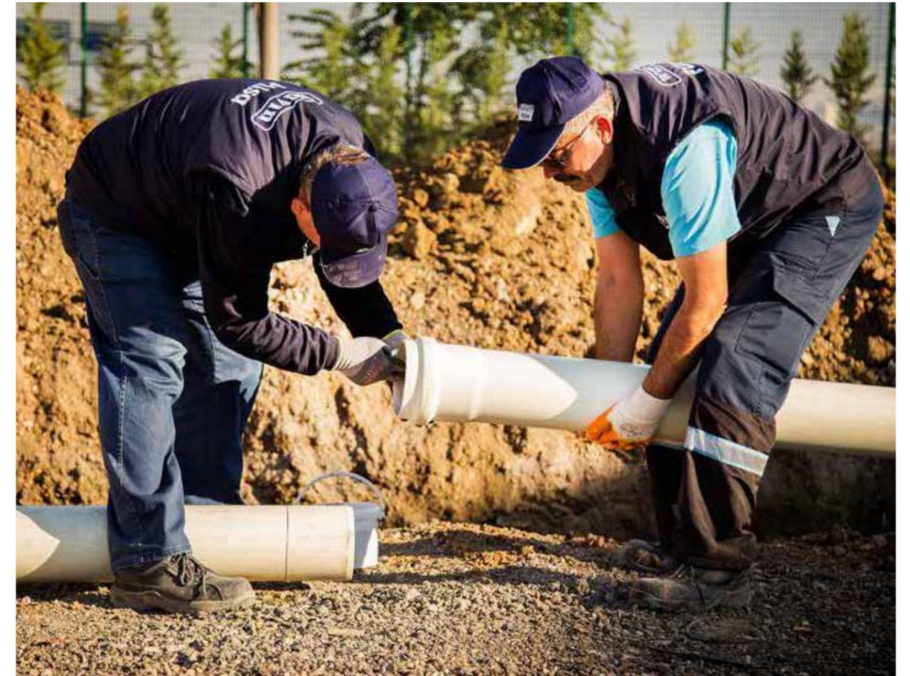
● The pipe joint with seal is made outside the excavation area and then the pipe can be carried to the excavation area. There is no need to make the welding in the excavation.
