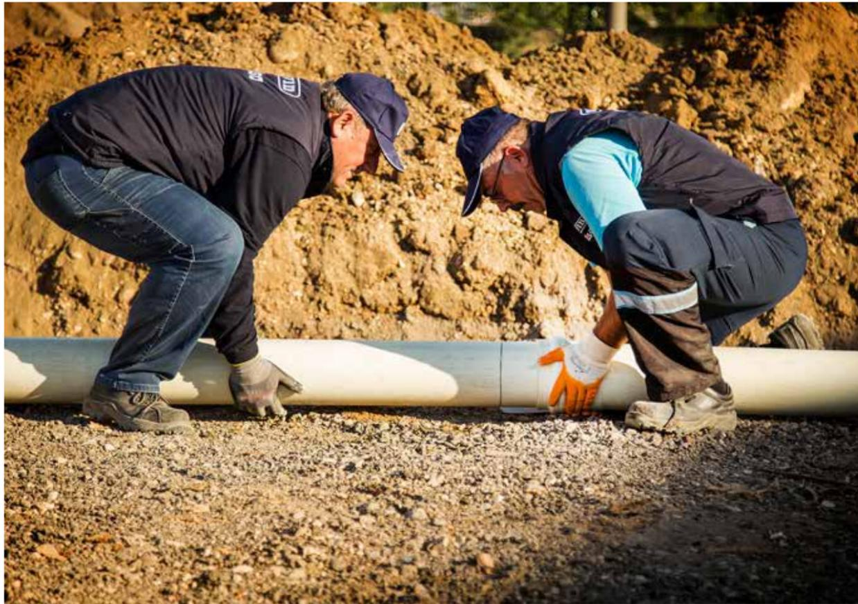
● Since it is not necessary to enter to the excavated pit, the width for burying the pipe may be narrower.
