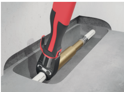
Fig. 30: Installation steps repair coupler.
