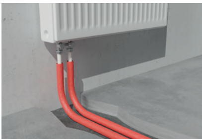
Fig. 48: Radiator installation examples with “Eurocone” screw connection.
